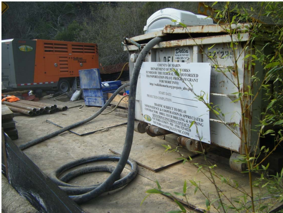
Photo 2. Project information board displayed for public viewing on Underhill Road.
