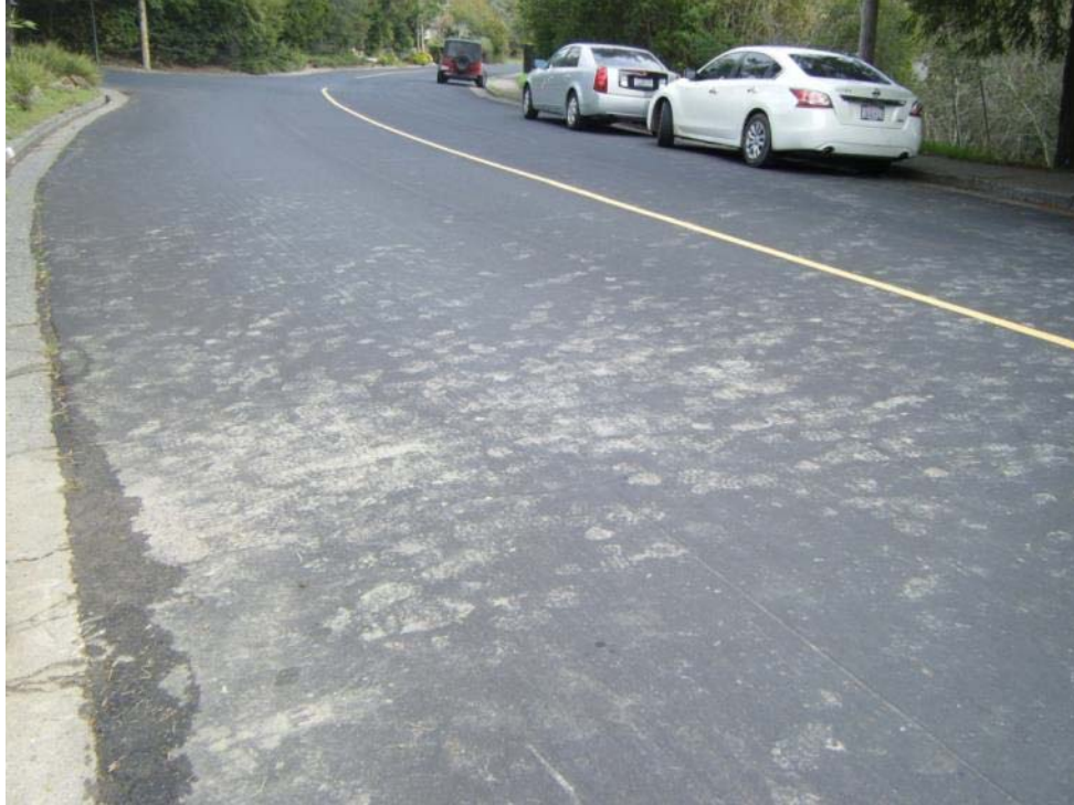
Photo 3. Boot washing needed to prevent tracking offsite.
