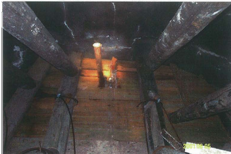
Figure 2-2: Top and Center of Timber Bulkhead
