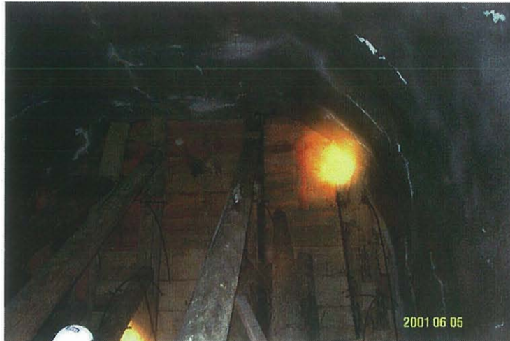
Figure 2-1. Timber Bulkhead at Face of Concrete Plug
