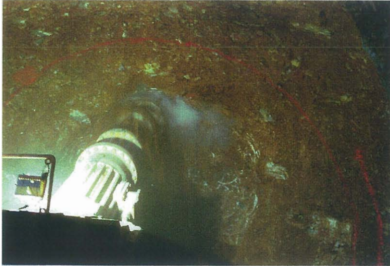
Figure 3-2. Roadheader Excavation in 3,000 psi Rock in Napa County
