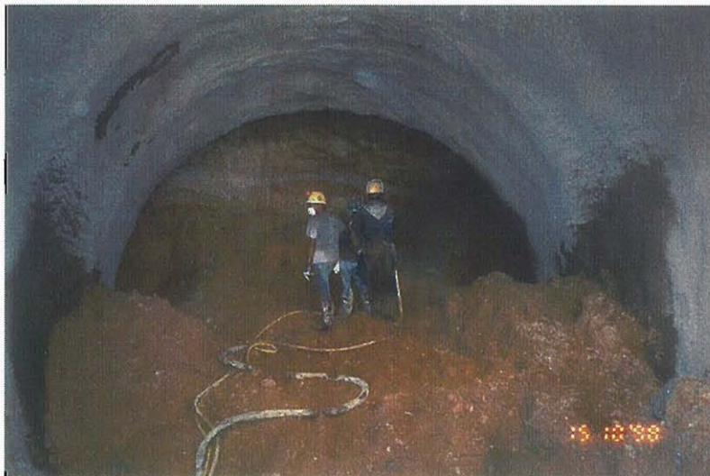
Figure 3-3. Typical Shotcrete Application in Tunnels
