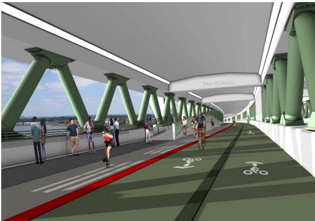
Figure 3: The proposed I-5 Bridge would include covered pedestrian and bicycle facilities, including a recreational multi-use pathway and directional bicycle commuter lanes.
