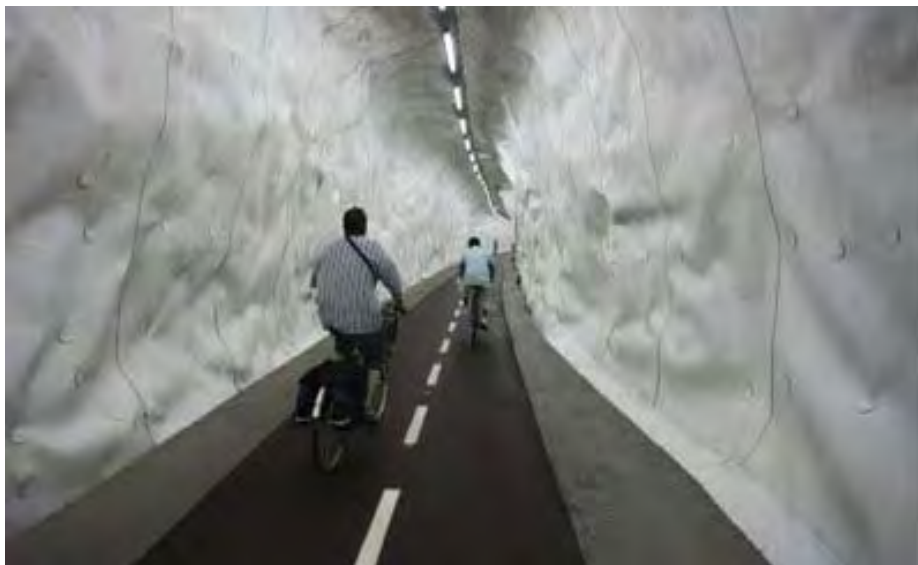
Photo 8-1: Example of similar bike/pedestrian tunnel in Spain
