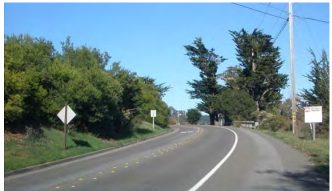
Photo 12-1 View north along segment 12a with shoulder on right side
