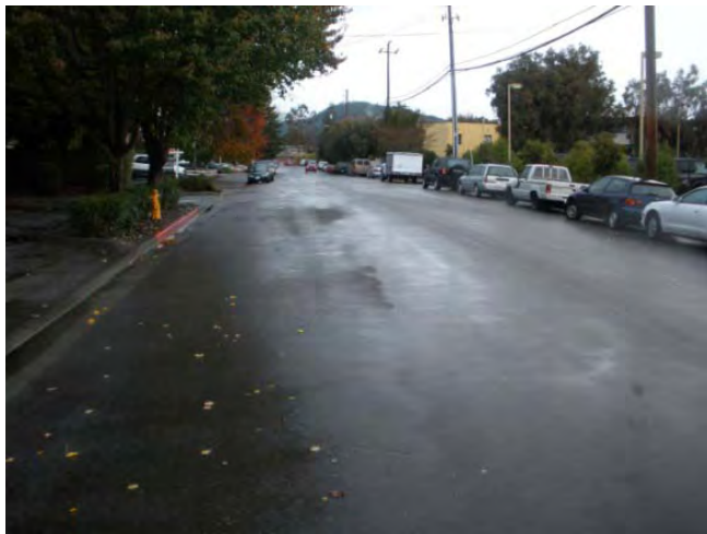
Photo 4-1 View north along Meadowsweet Drive near intersection with Laurel Drive.
