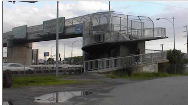
Nellen Avenue Overcrossing
